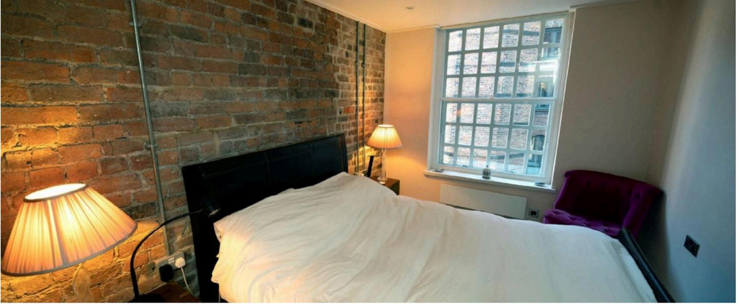
Discreet units with self-supporting panes. The tilt-in facility enables each secondary sash (panel) to be independently released from the outer frame and pivoted inwards through almost 180°.
